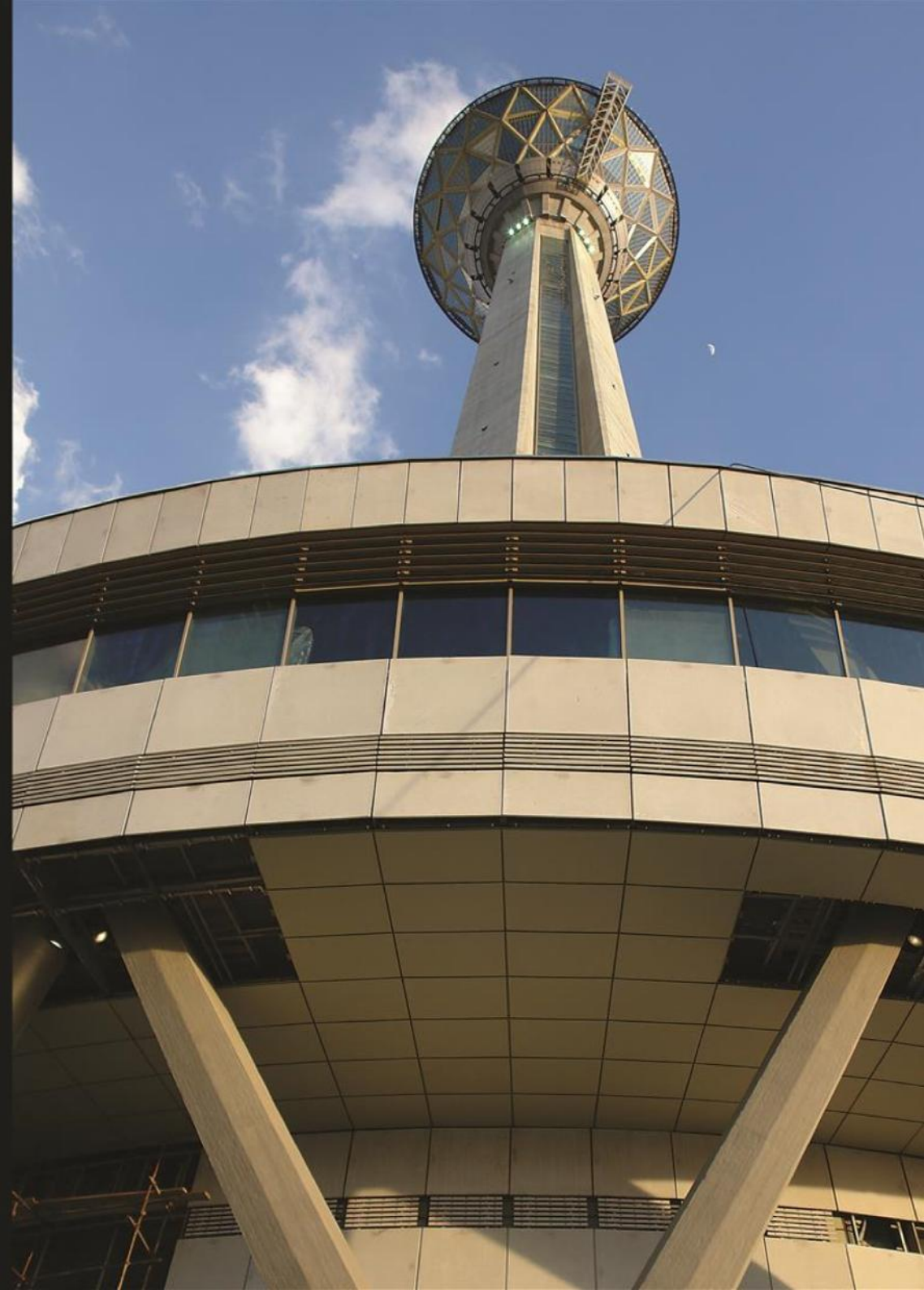
MILAD TELECOMMUNICATION TOWER
