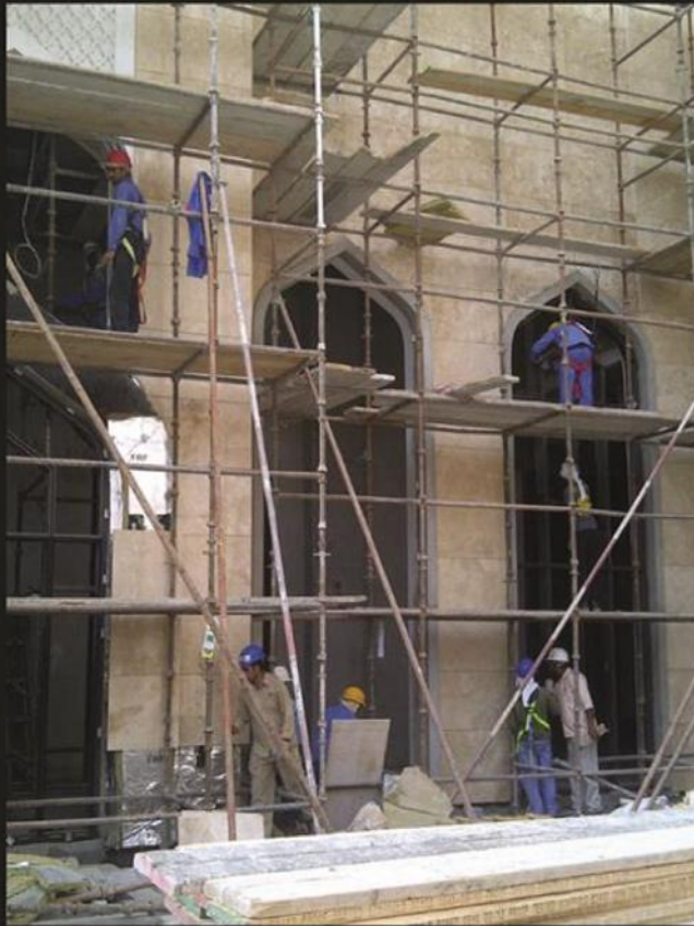
Ajman Saray Hotel, Travertine Installation
